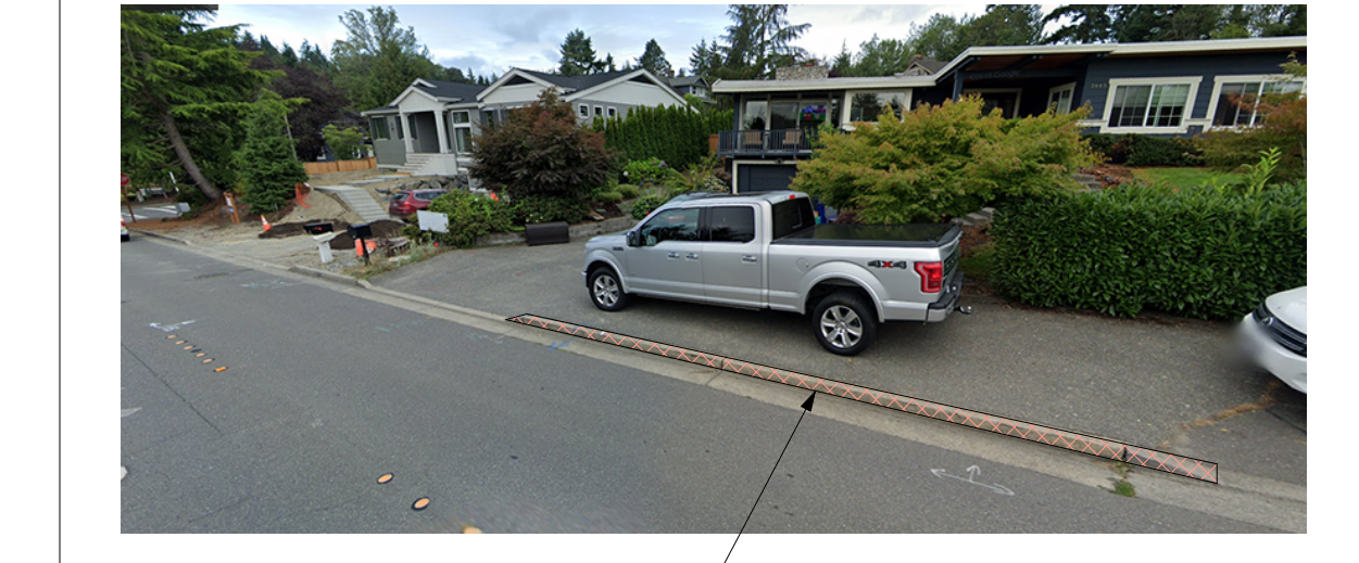
REMOVE UPPER PORTION OF VERTICAL CURB TO MATCH ADJACENT EXISTING MOUNTABLE CURBS. REGRADE SIDEWALK TO MEET NEW BACK OF CURB HEIGHT.
